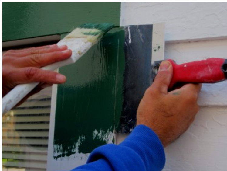
A VISTA member puts the finishing touches on window trim.
