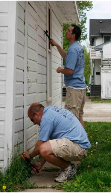
The longest yard: scraping the original paint off.
